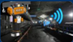
5G Tunneling preventive maintenance
